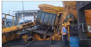
Installation, Commissioning and FAT
